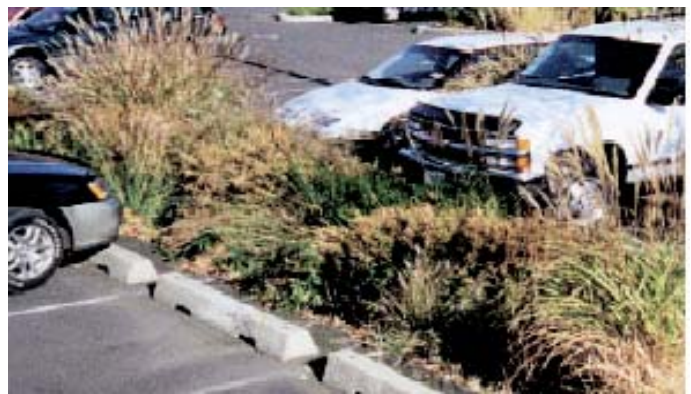
Swales in a parking lots can help filtrate runoff
